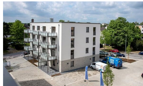
New construction in Hilden
